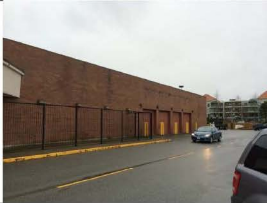
EXISTING ZELLER'S BUILDING - NORTH EAST CORNER ( PHOTO 6 )
