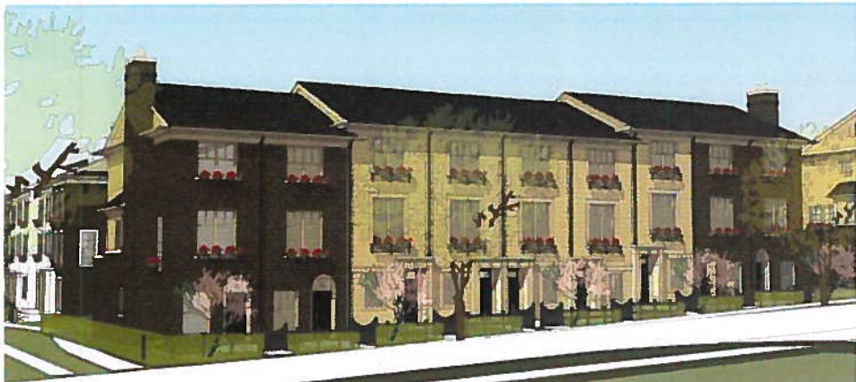
View of building 6 along 23A Avenue
