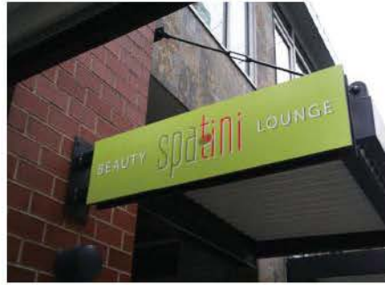
Sign cabinet with integral bracket and concealed electrical supply to building
