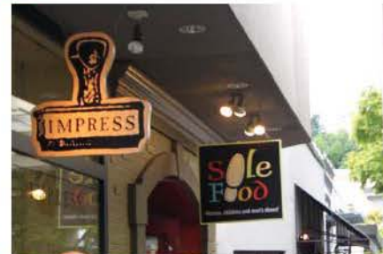
Unacceptable: externally illuminated sign face. Exposed suspension wire/ cables from canopy and poor example of exposed lighting.
