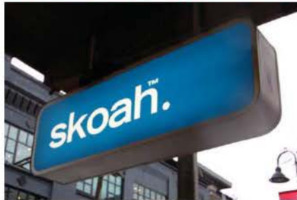
Unacceptable: Internally illuminated plastic face, back-lit "box" sign too thick and exposed electrical conduit to supply building.
