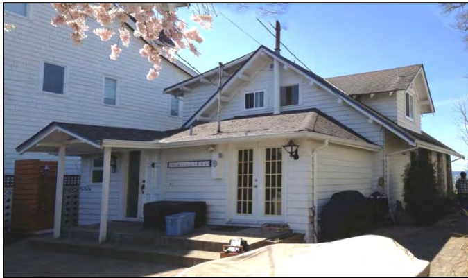
Photo 21: View from north east, note 1963 additions.
