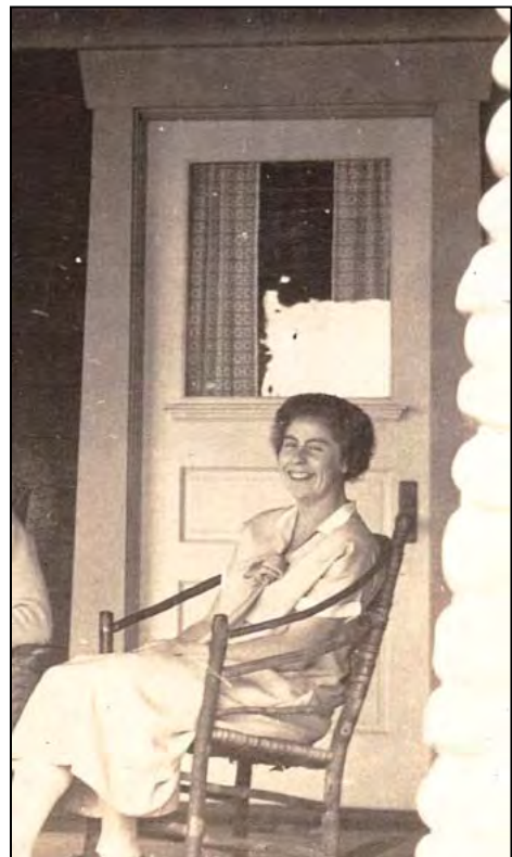
Photo 19: Original porch door.
