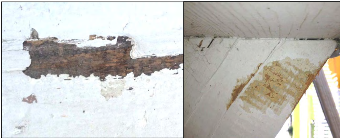
Photo 11: Original dark brown siding (left) & deep tan trimwork (right).
