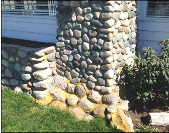
Photo 10: Detail of base of stone pier. Note later planter on left.
