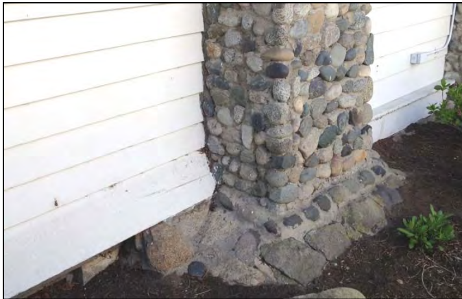
Photo 25: Typ. base of cobblestone pier, note wide flared bottom siding board.
