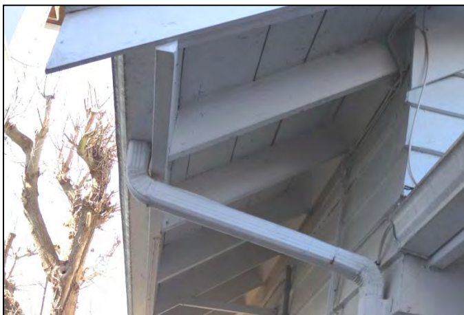
Photo 26: Typ. roof eave, note exposed rafter tails.
