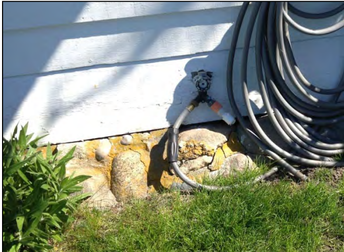
Photo 13: Original stone foundation. Note typical lichen growth.
