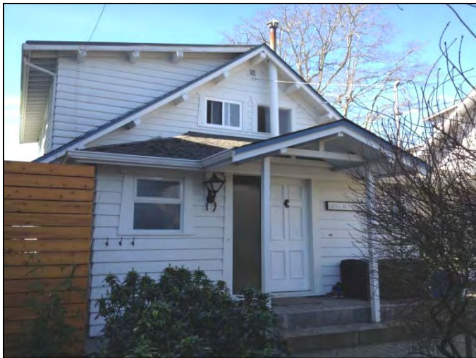
Photo 9: Rear of house showing 1963 additions.
