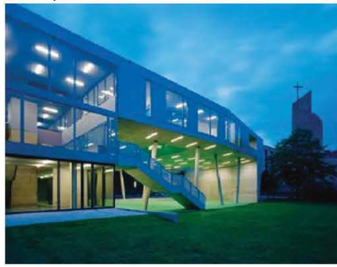
COLUMNS UNDER BUILDING
