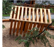
Hill Fort Method of Construction reference images above. Use of overlapping 4x4's fastened with threaded rod.
