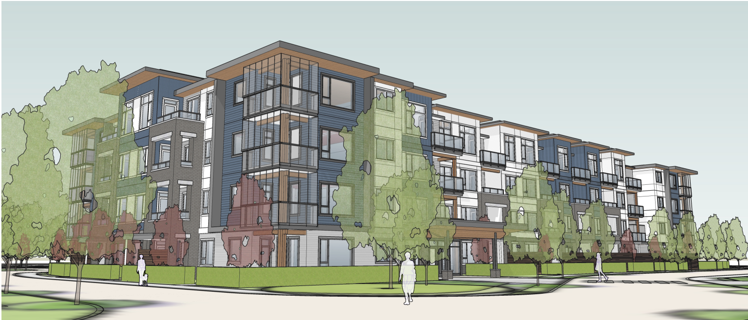
MIRRA 3: SOUTHWEST CORNER FROM 75A AVE.
