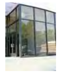
4 Storefront, Doors, And Windows: Tempered glass: clear with prefinished anodized black frame
