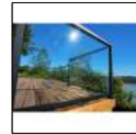
18 BLACK POWDER COATED ALUMINUM RAILINGS WITH CLEAR TEMPERED GLASS COLOR TO MATCH (BLACK OR SIMILAR)
