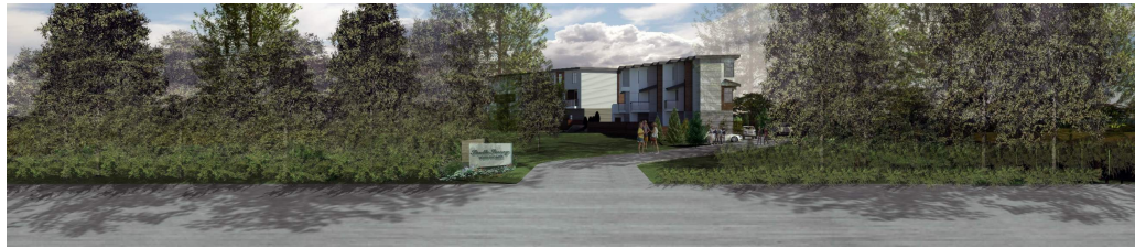
SITE ENTRANCE, 160 STREET
