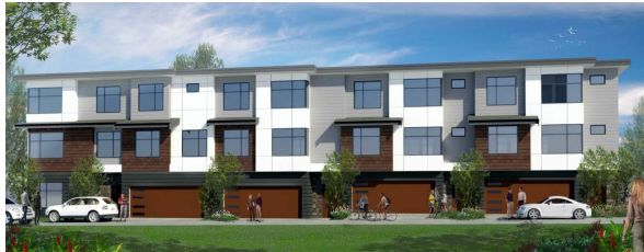
BLOCK-1, NORTH VIEW
