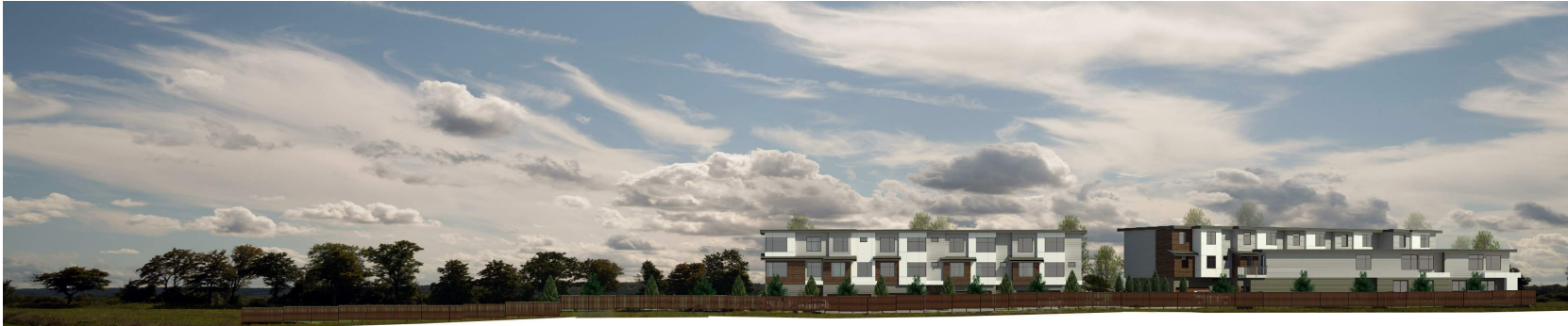
SITE NORTH VIEW
