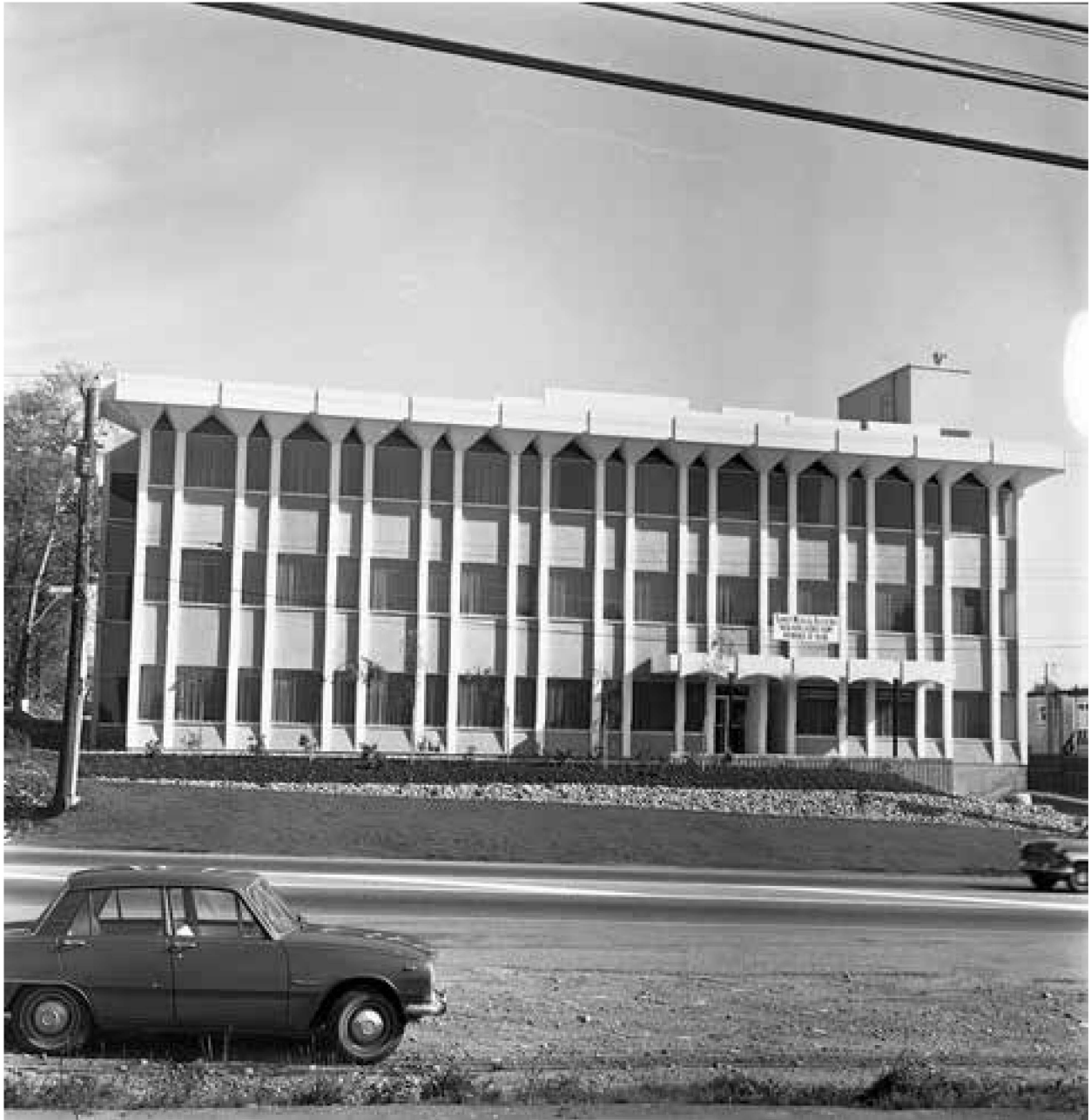
The new half-million dollar medical centre built by North Surrey doctors on King George Highway north of 96th Avenue, October 16, 1969 [Surrey Archives 1992.036.16786 & 16787]
