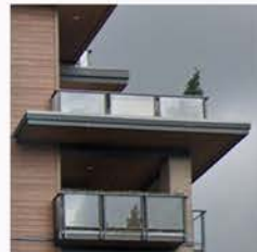
03 GUARDRAIL & METAL FACIAL AT BALCONY
