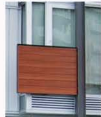
COMPOSITE PANEL WITH METAL FRAME
