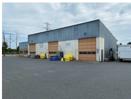
3 - 1 STOREY BUILDING - NORTH VIEW
