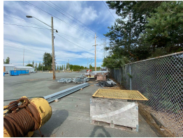
7 - EQUIPMENT AND STORAGE ON SITE
