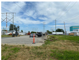
5 - EQUIPMENT AND STORAGE ON SITE
