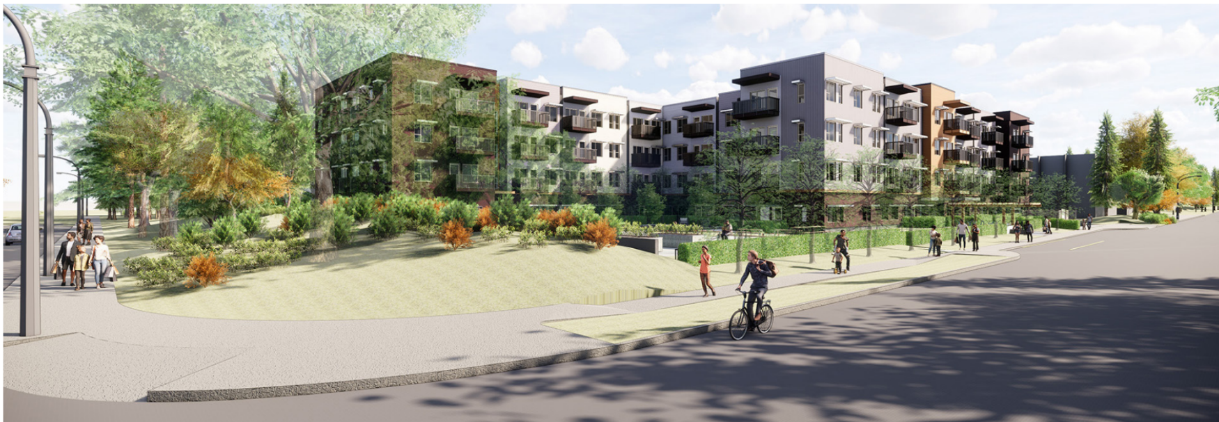
1- VIEW FROM INTERSECTION OF 152ST AND 99AVE
