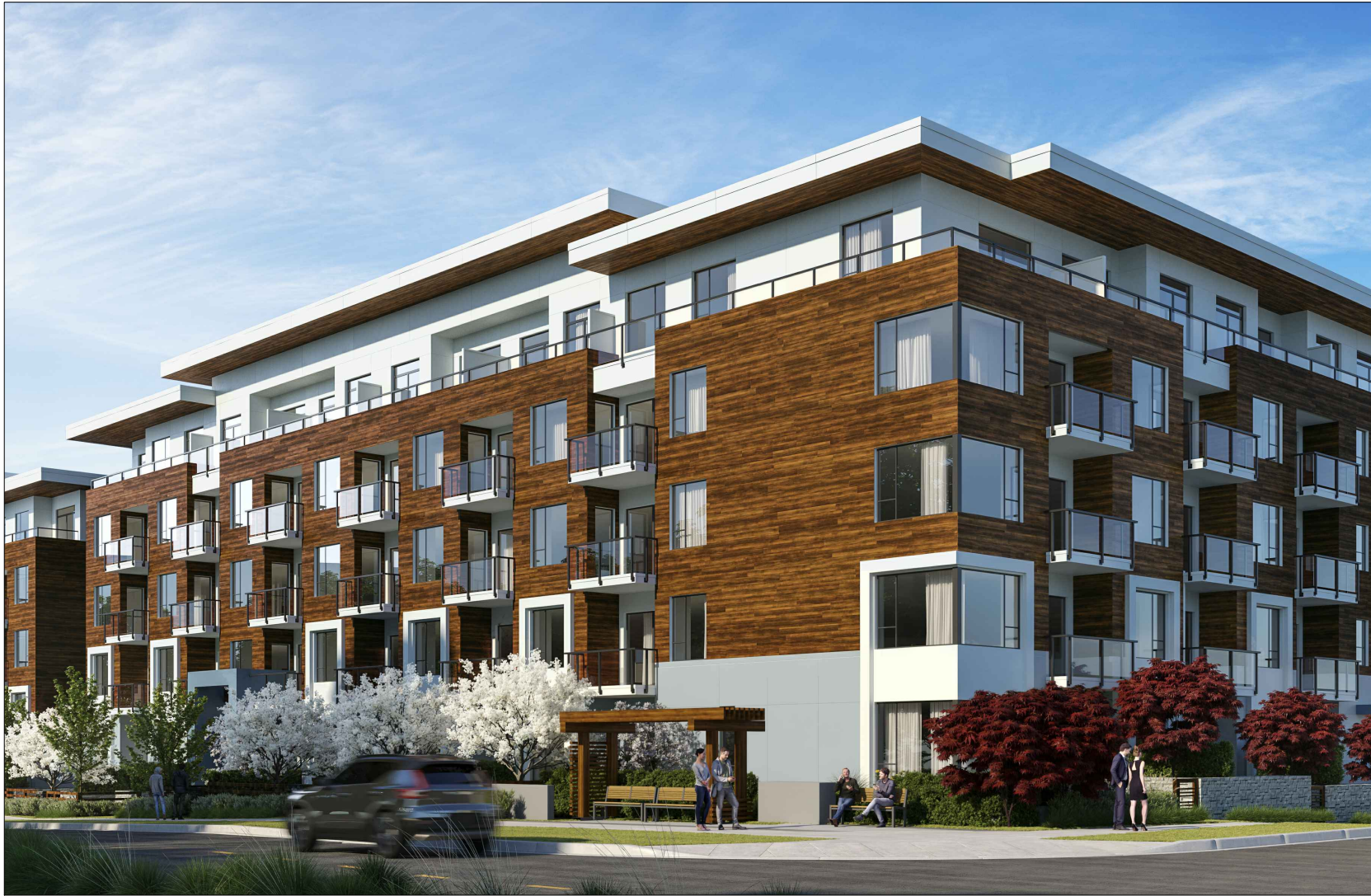
VIEW FROM SOUTHWEST
