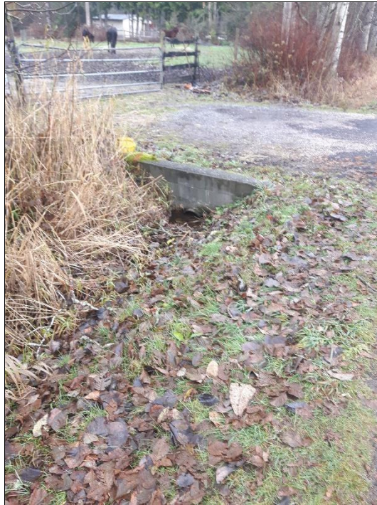
Photograph 5: 48 th St. Ditch at Home Plate (east view)
