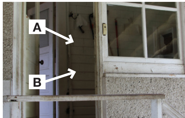
Localized areas showing surviving original wood cladding: cedar shingles (A) and shiplap siding (B).
