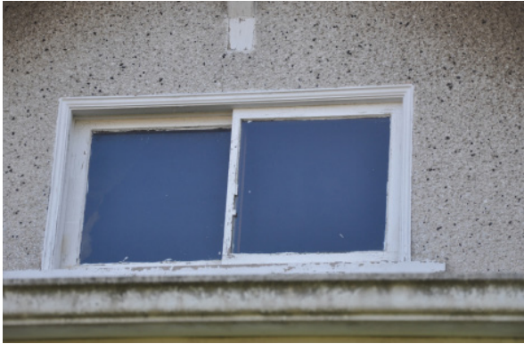
Clear, sliding wood window assembly at front gable wall (attic).
