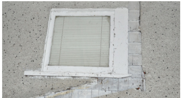
Fixed wood window at rear (east) elevation). Note exposed original wood window exterior casing, which would have been a typical trim detail for all window openings.
