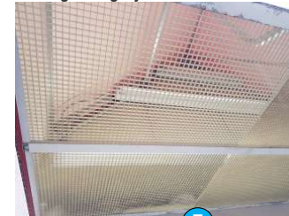
Existing Awing System
