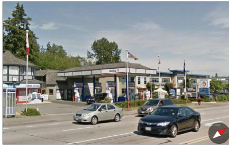
S5. EXITING SERVICE STATION LOCATED ON PROJECT SITE NORTH OF PROPOSED BLDG (128ST)
