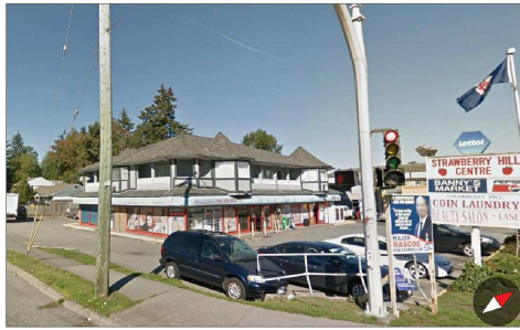
S4. INTERSECTION OF 128ST & 76 AVE EXISTING MIXED-USE BLDG ON PROJECT SITE
