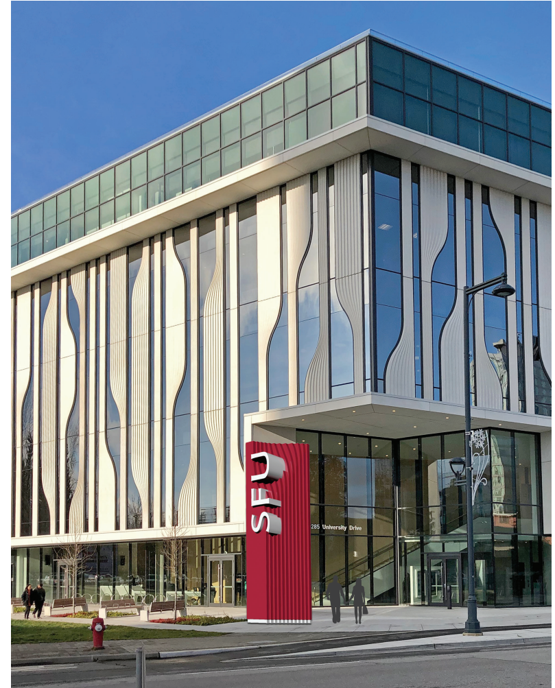
View of building entrance from corner of University Drive & 102A Avenue.
