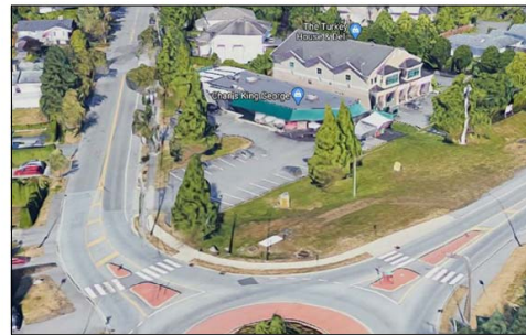
A3. AERIAL VIEW FROM TRAFFIC CIRCLE
