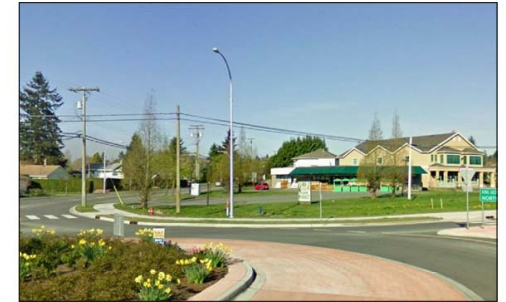
S2. NW VIEW FROM TRAFFIC CIRCLE
