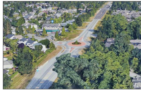
A1. AERIAL VIEW NW - KING GEORGE BLVD
