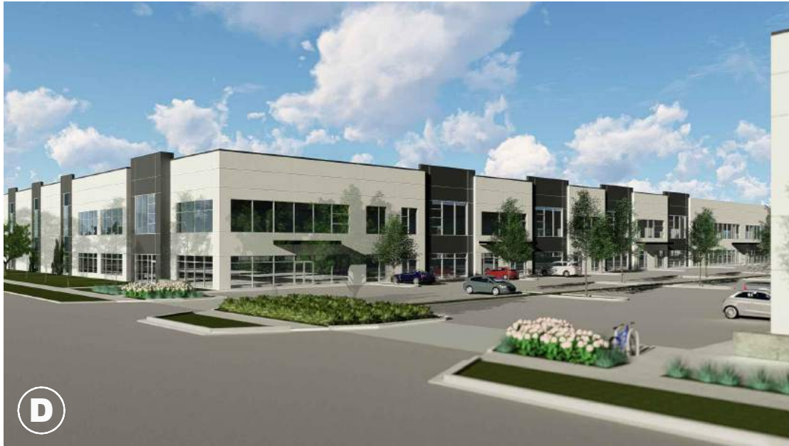
BUILDING D - VIEW TO THE SOUTH WEST
