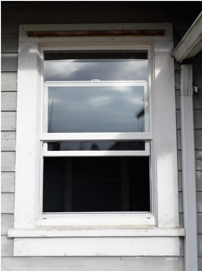
Figure 81: W-02 Front of cottage double-hung window
