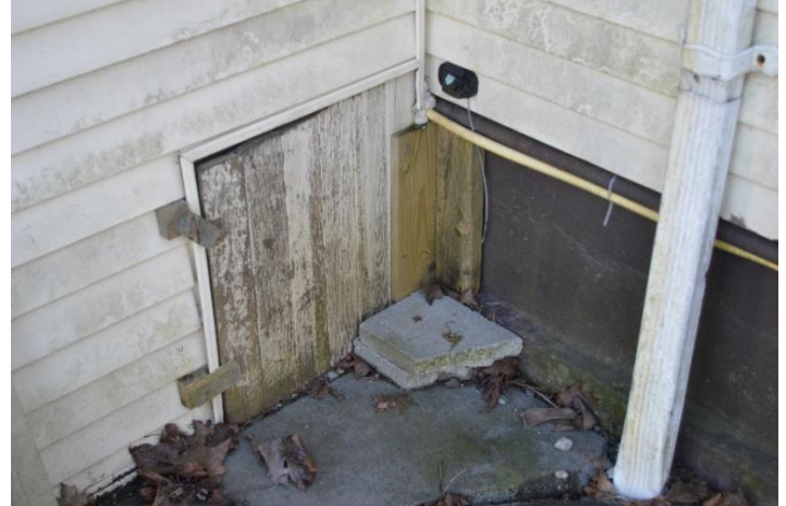
Figure 17: Crawl space access half door
