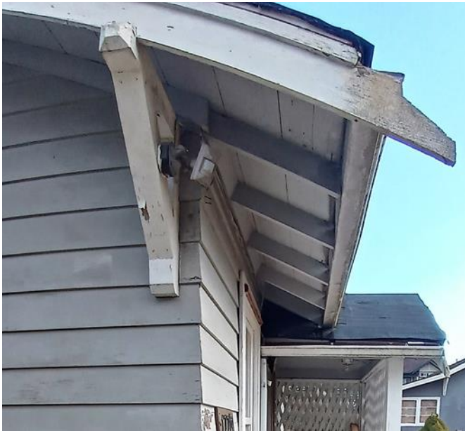
Figure 73: Exposed rafters, bargeboard tail, and knee-bracket
