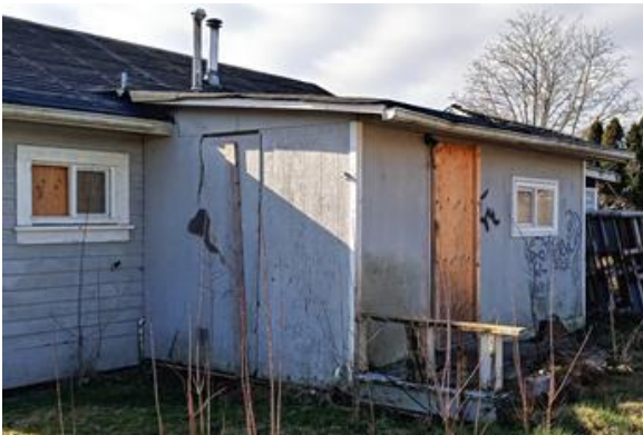
Figure 64: Plywood addition on the back of the cottage
