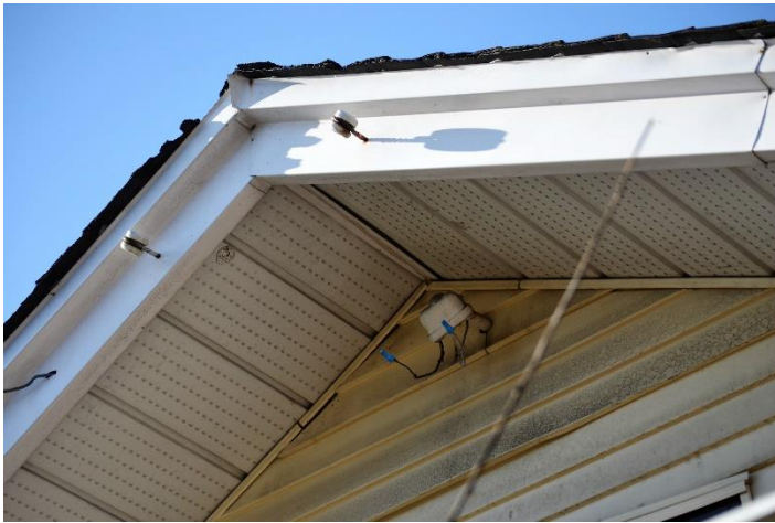
Figure 20: Gable end with closed perforated aluminum soffit
