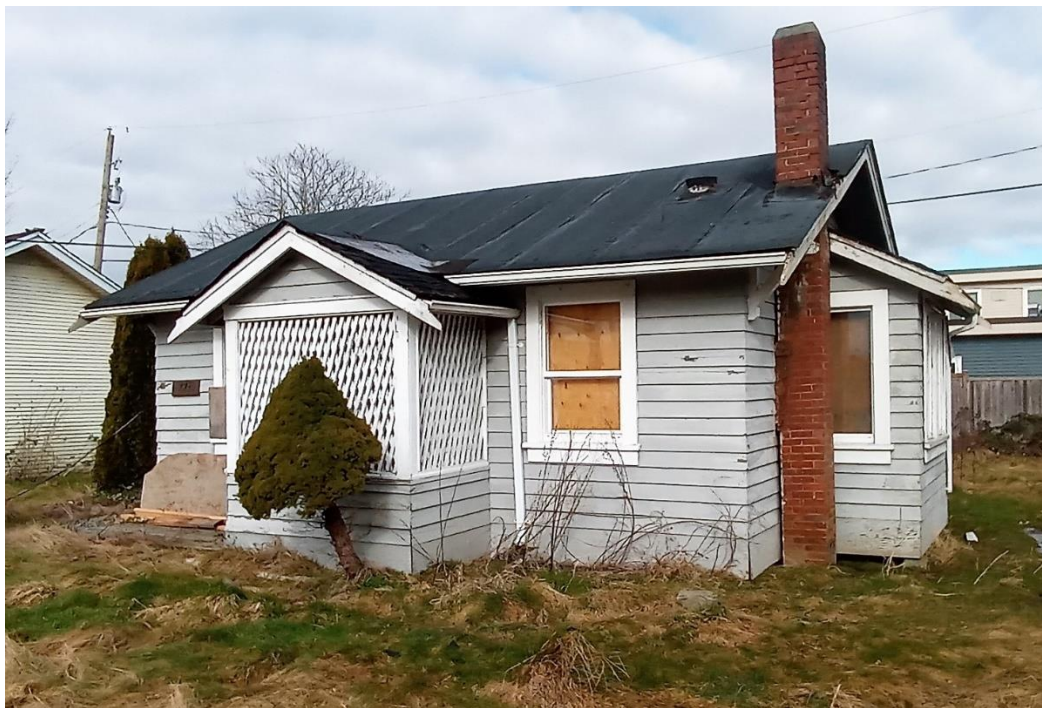
Figure 62: Northeast corner of the Mooring Cottage
