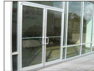
STOREFRONT ALUMINUM FRAMED WINDOWS & DOORS COLOUR: NOT APPLICABLE - REFER TO PAINT COLOURS ELEVATIONS FINISH SCHEDULE NO: 6
