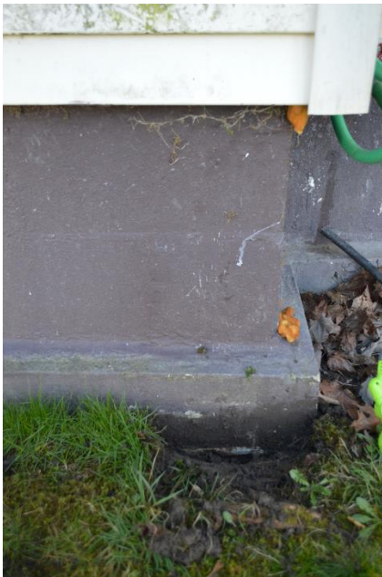
Figure 18: Depth of concrete footing
