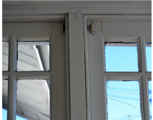
Figure 34: Interior view of W-05
