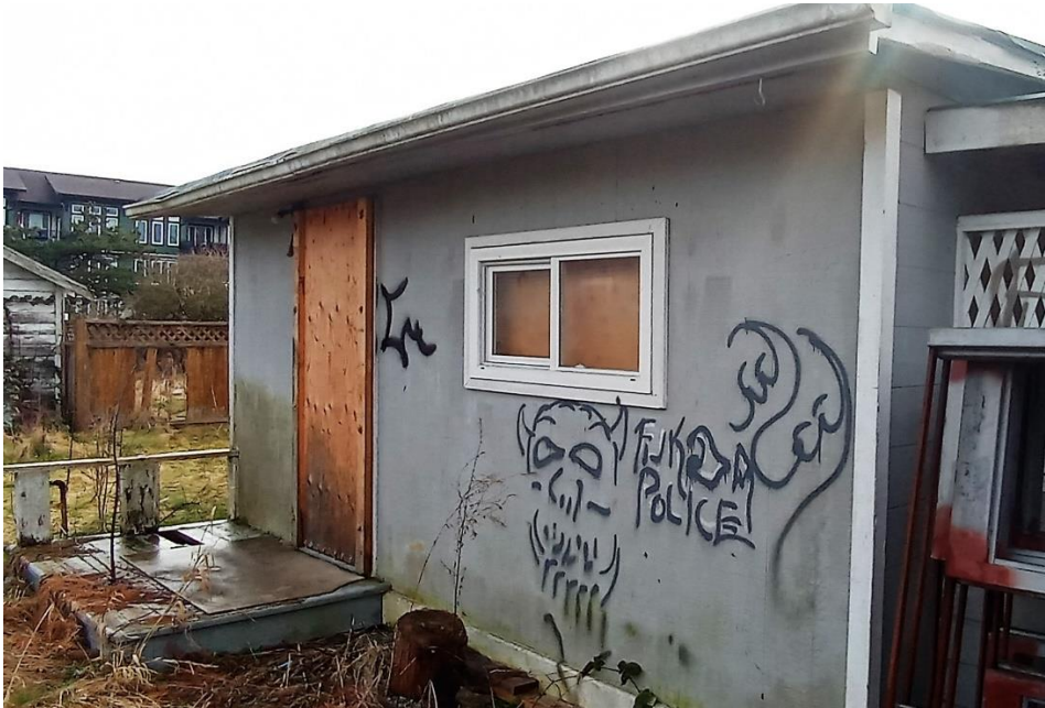
Figure 91: Plywood addition with PVC slider window
