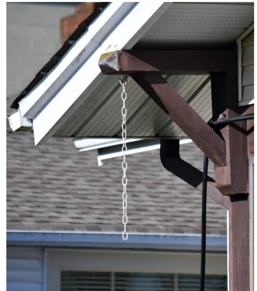
Figure 24: Knee-bracket with pointed end at southwest corner of front porch
