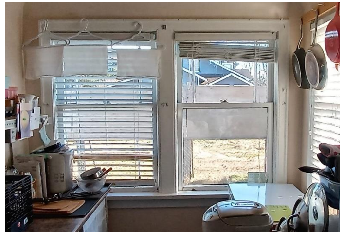
Figure 36: Interior view of W-14-15
