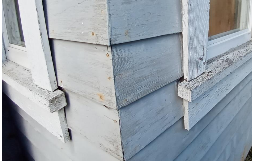
Figure 78: Tapered siding corner
