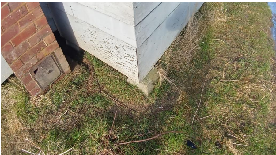
Figure 69: Concrete block footing next to chimney foundation
