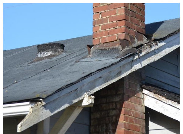
Figure 76: Tar paper roofing and chimney flashing
