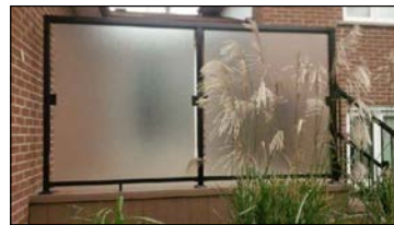
POWDER COATED ALUMINUM PRIVACY SCREENS BLACK ALUMINUM WITH OBSCURED TEMPERED GLAZING ELEVATIONS FINISH SCHEDULE NO: 10
