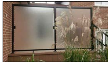
POWDER COATED ALUMINUM PRIVACY SCREENS BLACK ALUMINUM WITH OBSCURED TEMPERED GLAZING ELEVATIONS FINISH SCHEDULE NO: 10
