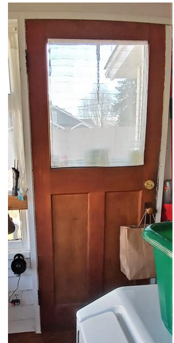
Figure 51: Exterior back door inside
