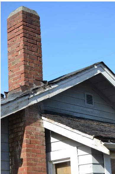
Figure 88: Brick chimney adjacent to ding nook
