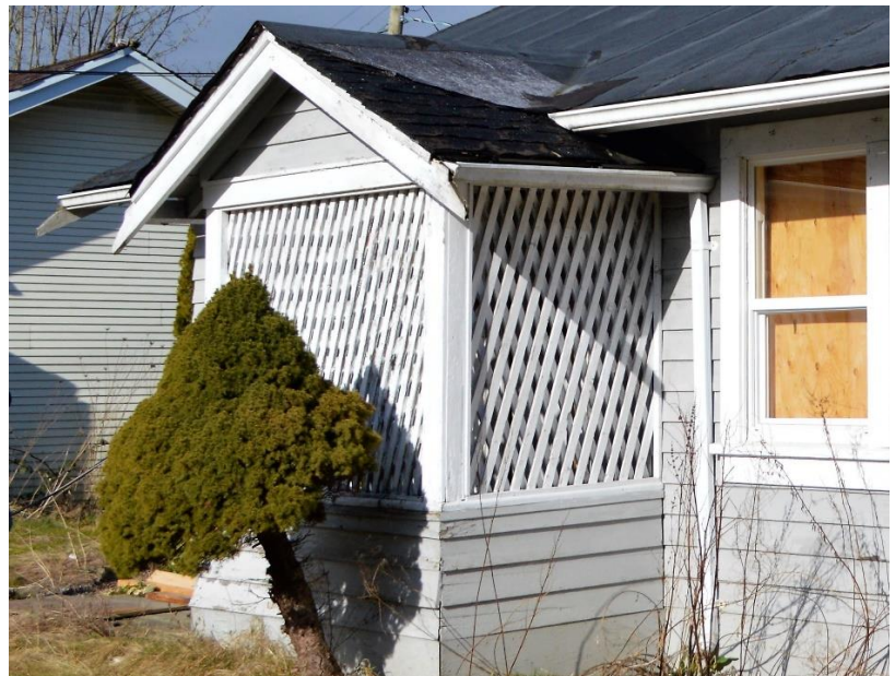
Figure 80: Front porch lattice screen
