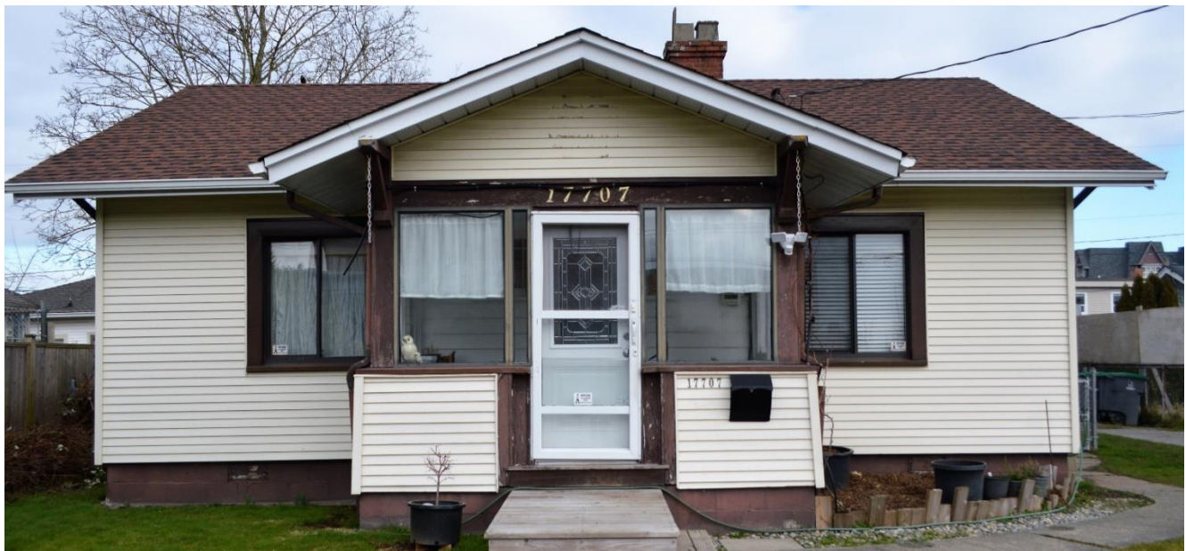
Figure 15: Front elevation showing low pitch roof, the generous overhang, symmetrical façade, and central front porch
