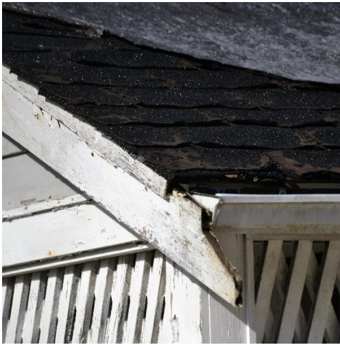
Figure 71: Tar paper on top of asphalt shingles
