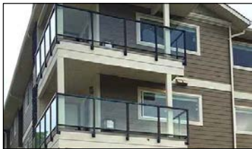
POWDER COATED ALUMINUM GUARDRAILS WITH TEMPERED GLAZING PANELS BLACK ALUMINUM WITH CLEAR TEMPERED GLAZING ELEVATIONS FINISH SCHEDULE NO: 7
