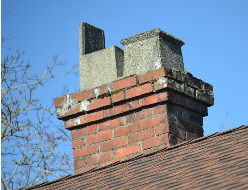
Figure 52: Exposed chimney shaft viewed from 56A Avenue
