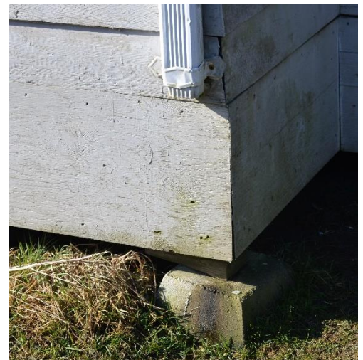
Figure 70: plywood base board and block footing
