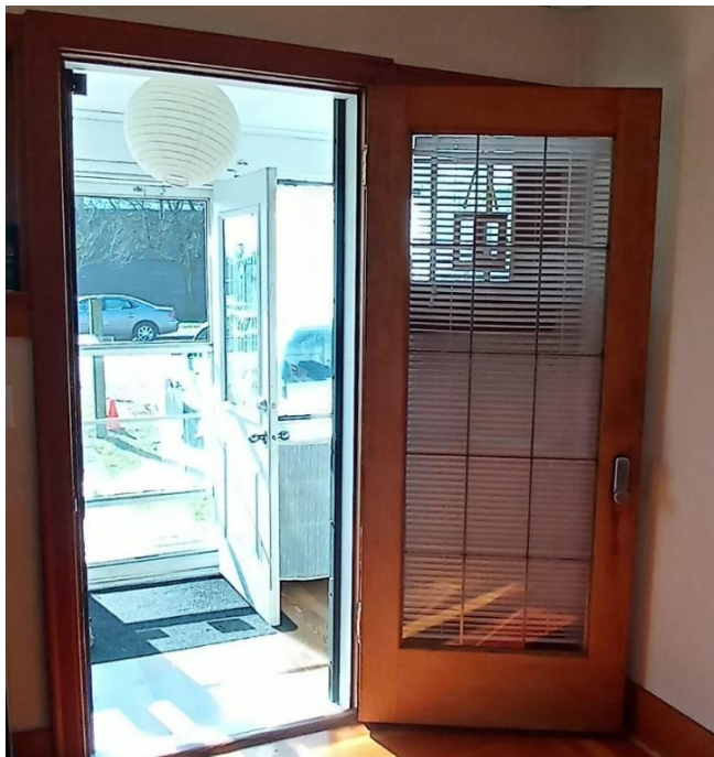
Figure 49: Interior front door
