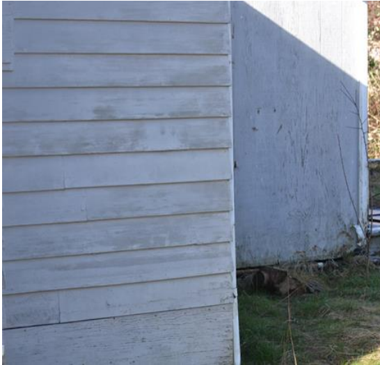
Figure 77: Typical lap siding with plywood addition behind
