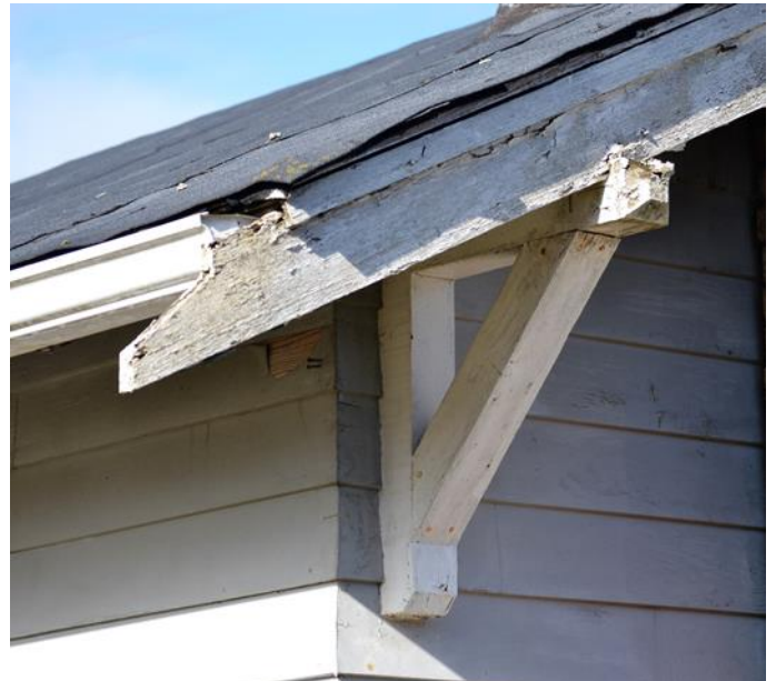
Figure 74: Tar paper roofing, bargeboard, and knee-bracket
