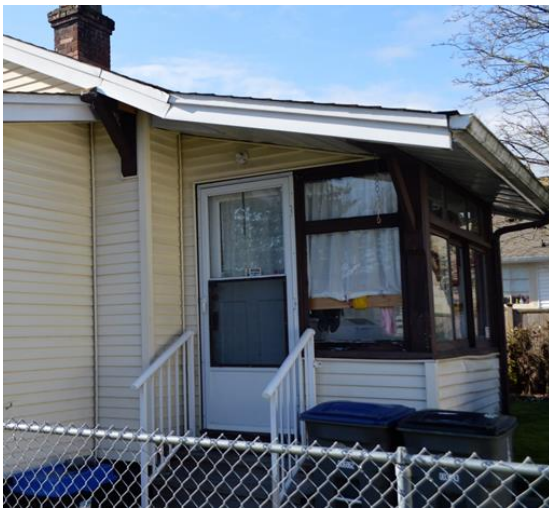
Figure 30: Enclosed back porch with shed roof
