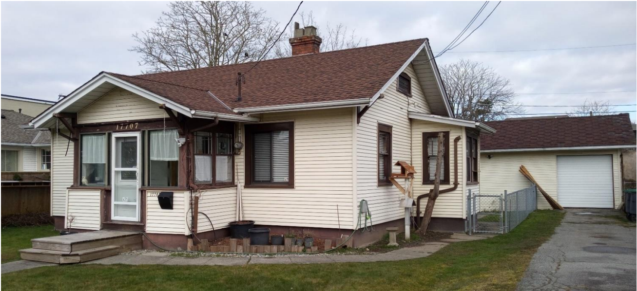
Figure 9: The Mooring House view of northeast corner with the garage at the back
