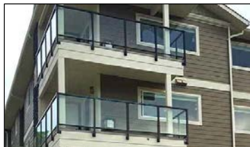
POWDER COATED ALUMINUM GUARDRAILS WITH TEMPERED GLAZING PANELS BLACK ALUMINUM WITH CLEAR TEMPERED GLAZING ELEVATIONS FINISH SCHEDULE NO: 7
