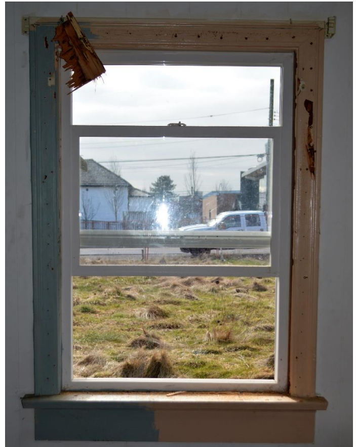
Figure 82: W-02 Interior face of double-hung window
