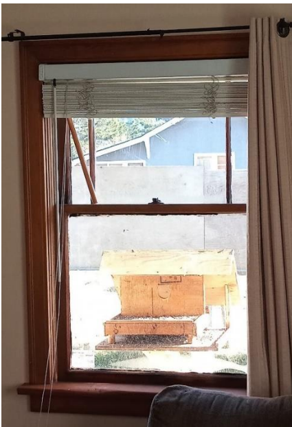
Figure 41: W-117 interior view
