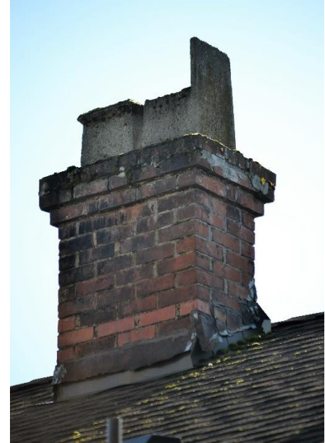
Figure 53: Exposed chimney shaft viewed from the backyard
