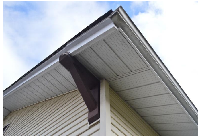
Figure 21: Wooden knee bracket northeastern roof corner
