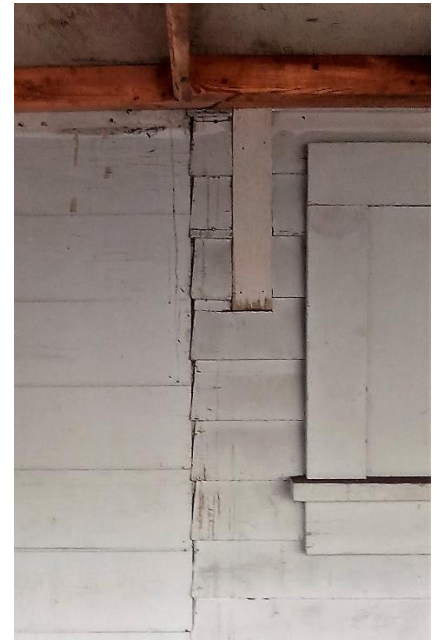
Figure 92: Change of siding on west wall
