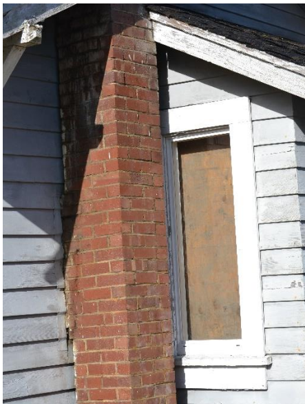
Figure 89: Chimney in front of window
