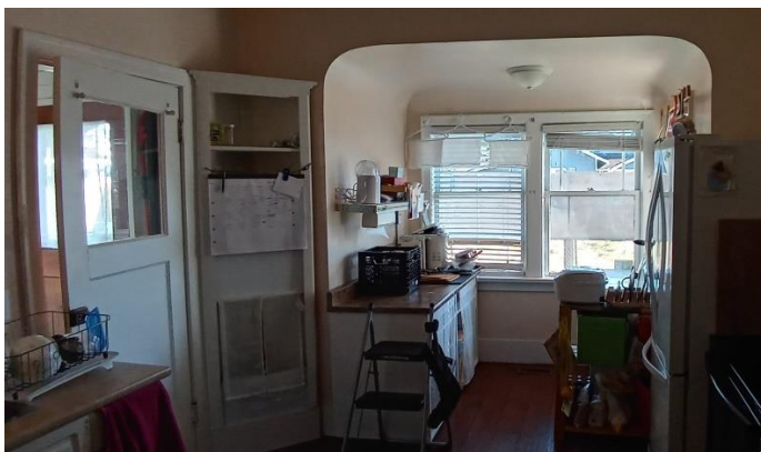
Figure 54: Dining nook interior framing and interior back porch door
