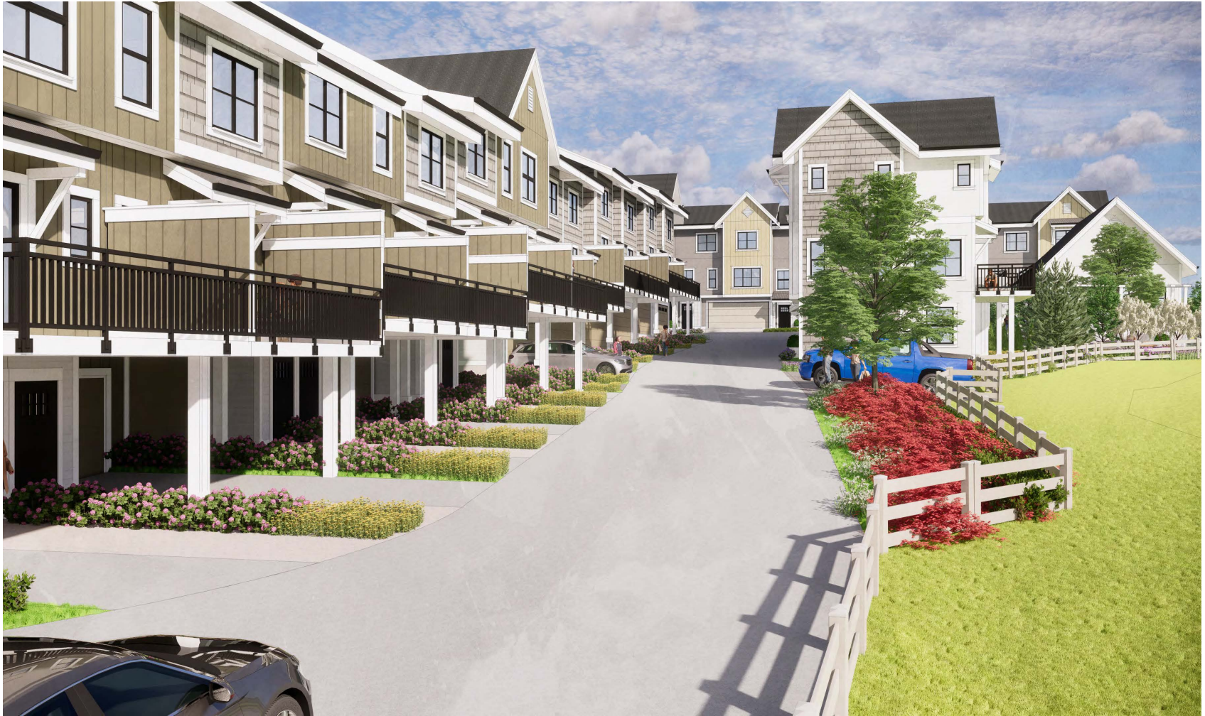
VIEW LOOKING SOUTH ALONG EAST LOT
