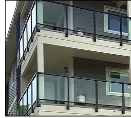
POWDER COATED ALUMINUM GUARDRAILS WITH TEMPERED GLAZING PANELS DARK GRAY ALUMINUM WITH CLEAR GLAZING ELEVATIONS FINISH SCHEDULE NO: 13
