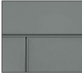
PREFINISHED FIBRE-CEMENT PANELS C/M FRY REGLET TRIMS COLOR: "GREY PENNANT A2000" ELEVATIONS FINISH SCHEDULE NO: 2
