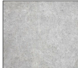
EXPOSED CONCRETE FOUNDATION WALLS
