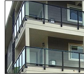
POWDER COATED ALUMINUM GUARDRAILS WITH TEMPERED GLAZING PANELS
