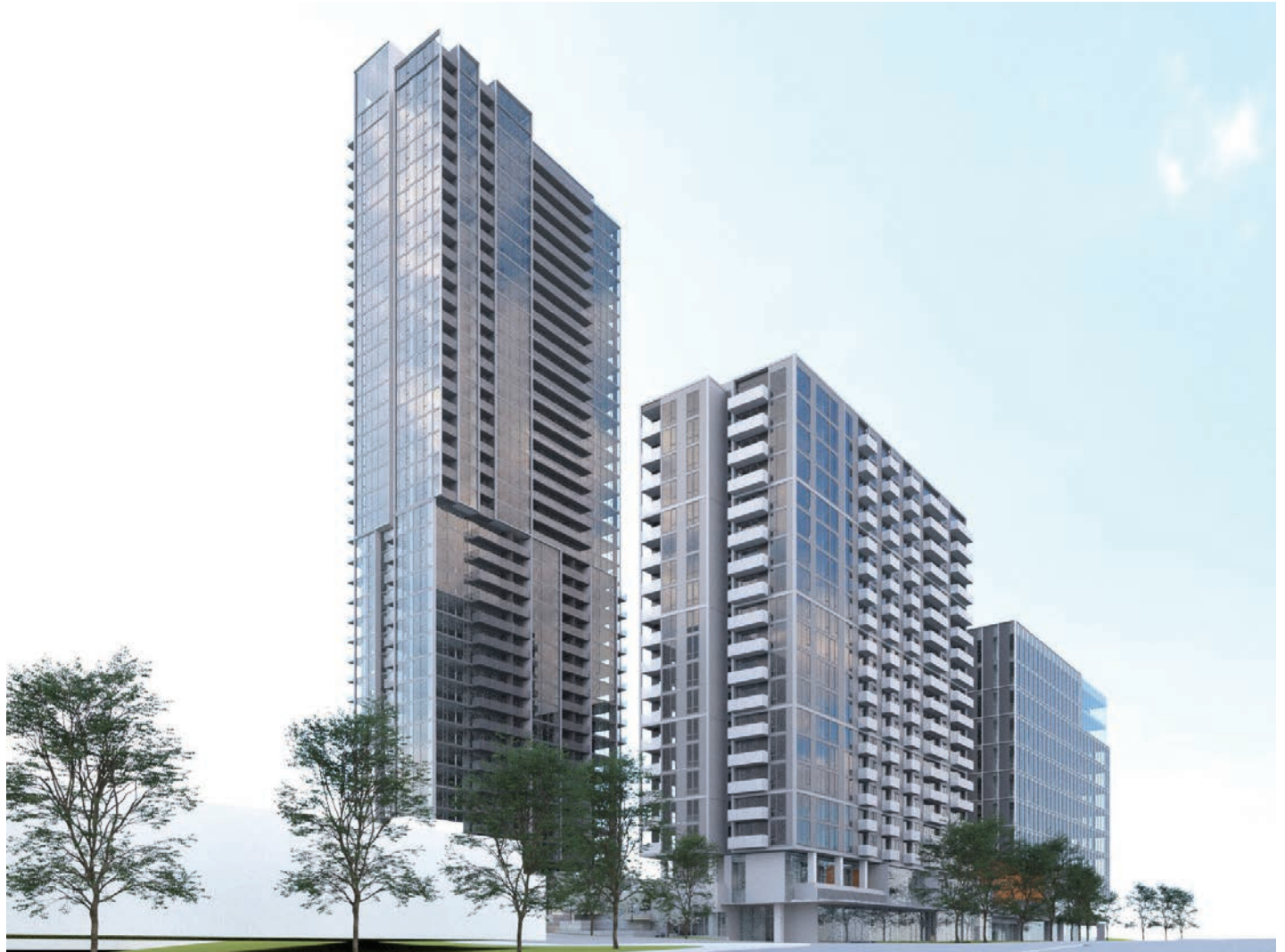
SE CORNER ALONG KING GEORGE BLVD
