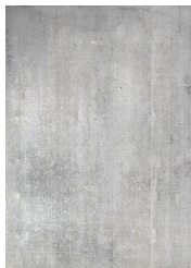
CONCRETE COLUMNS AND WALLS
