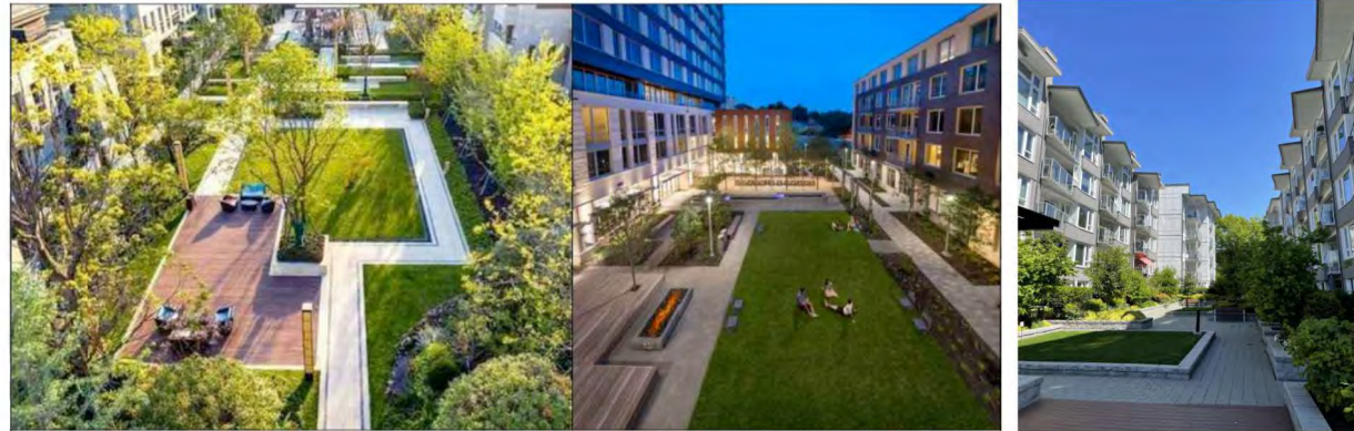
A good mix of hard and soft landscaping choices at the mews and courtyards will give this node a strong residential feel. These additional spaces for gathering and interaction foster healthy community development.
