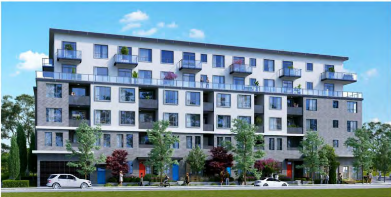
A mix of brick, metal, and fiber cement materials, along with varying building heights will provide this node with a more residential feel throughout. Two-storey townhouse expressions will be provided to ground the buildings and enhance the pedestrian experience along road frontages.
