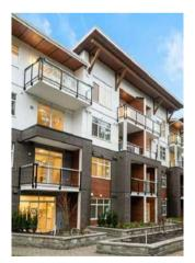
Two storey elements are used to connect the building with the street and to create rhythm to the horizontal north facade.
