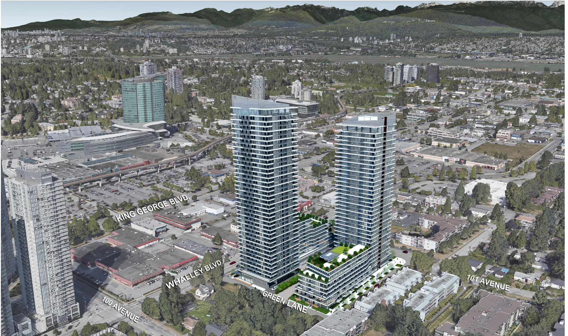
CONTEXT VIEW FACING NORTHWEST & SURREY CITY CENTRE
